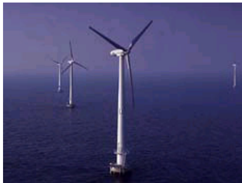
Figure 1-9. Vindeby Offshore Wind Farm. From www.windpower.org (1997) © Bonus.
