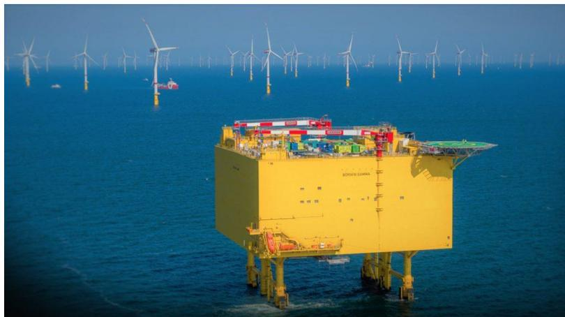
Figure 50 : Station de conversion en mer, BorWin gamma tenneT, source [54]
